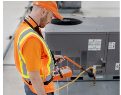
Inspecting for gas indications
