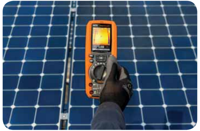
PV field thermography.
